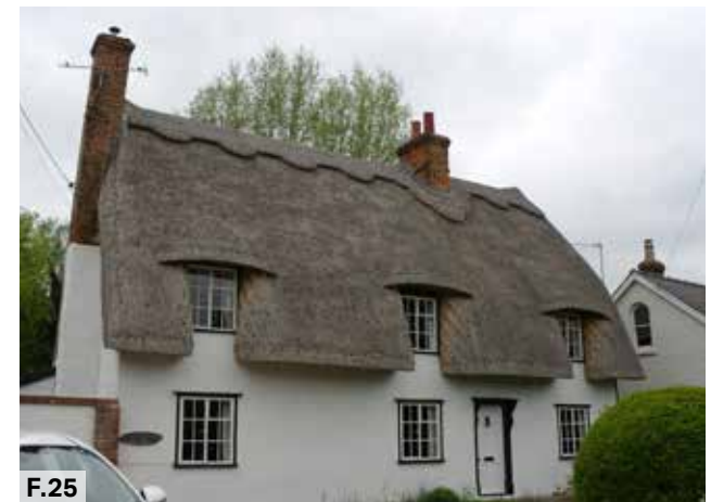
Figure 25: 1.5 storey cottage with dormer windows.
